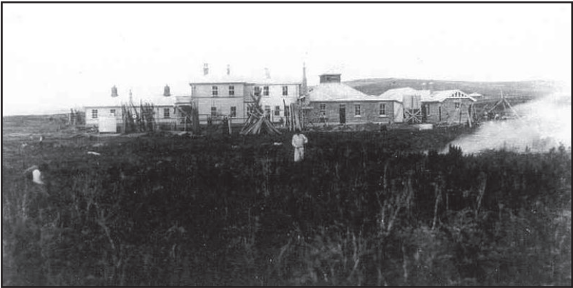
Figure 2: Tokanui Hospital buildings, January 1915, unoccupied. This image of Tokanui shows men digging drains.
